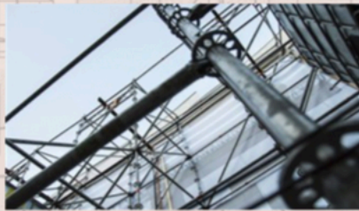
SWING STAGE - REPEL - SCAFFOLDING
